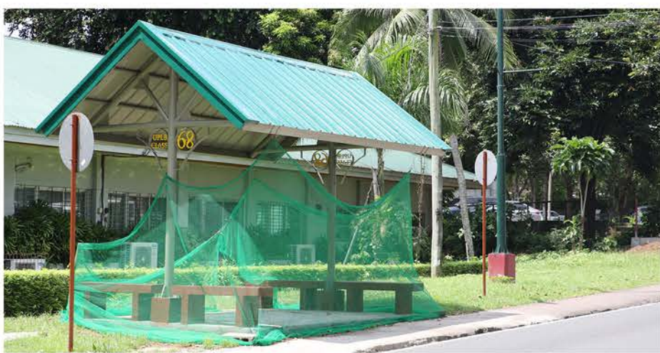
SHIELD FROM RAIN OR SUN. Located across the Christian School International is one of the six waiting sheds that the UPCA Class ‘68 has constructed in the campus. (Photo by VRManingas/OPR)
